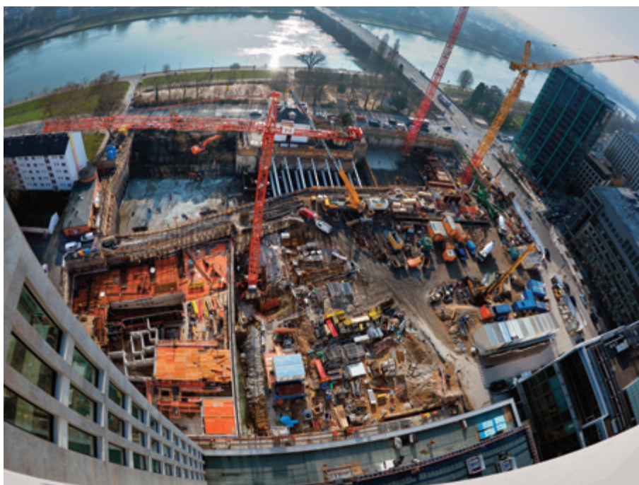
Current MainTor site under construction
