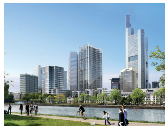
Frankfurt, MainTor project
